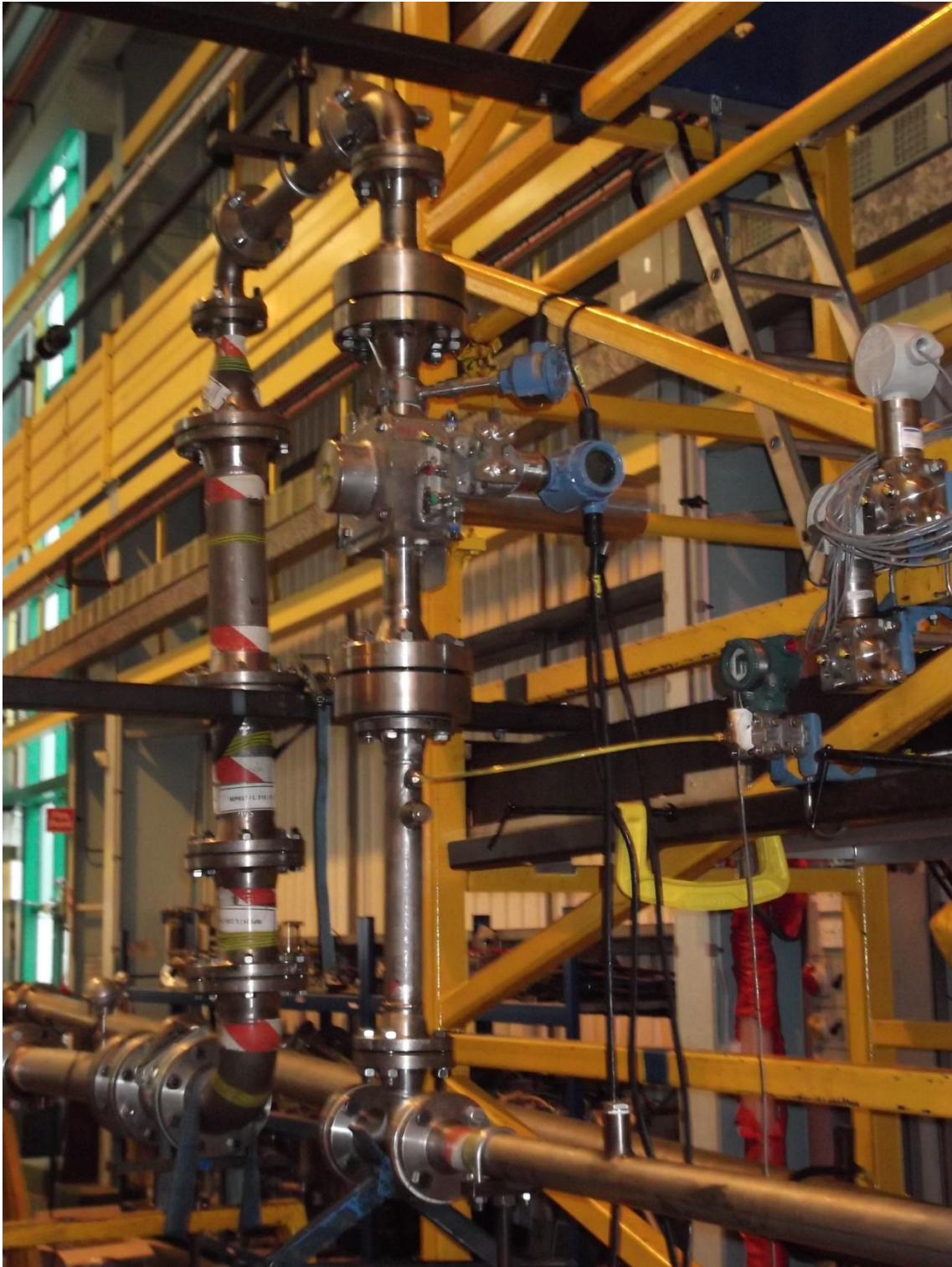
Figure 2: View Showing 2-inch SP MPFM Installation in Facility Test Section.
