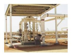
Bulk meters are large size Multiphase flow meters with sizes ranging up to 24 Inch with measurement capability of up to 500,000 BPD.
